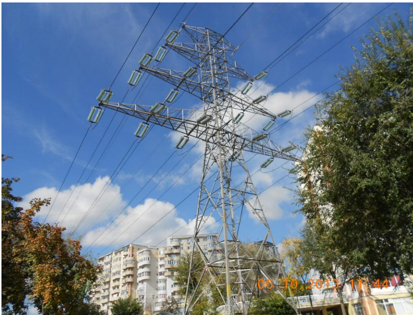
Fig. 1.7 - 110 kV pole with 4 circuits
