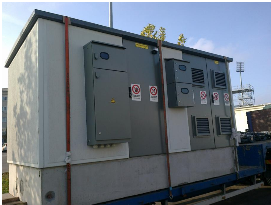
Fig. 1.11 - Enclosed 1.2 MVA MV/LV substation [webSUP]
