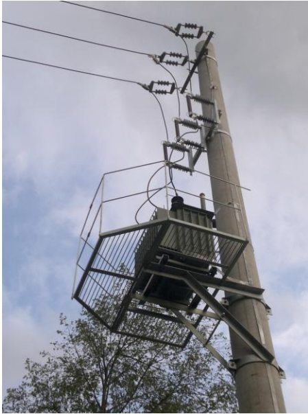
Fig. 1.9 - MV concrete pole and outdoor MV/LV substation
